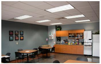
Office space before and after T8 fluorescents were replaced with **X-Series LED T8** tubes. 15 watt X-Series tubes are a direct replacement for 32 watt fluorescents.
